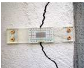
Installation Rissmonitor
